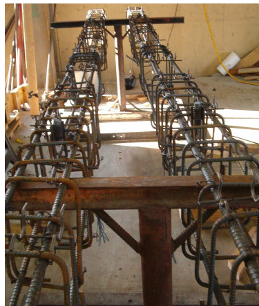
Figure 6: Rebar Cages
