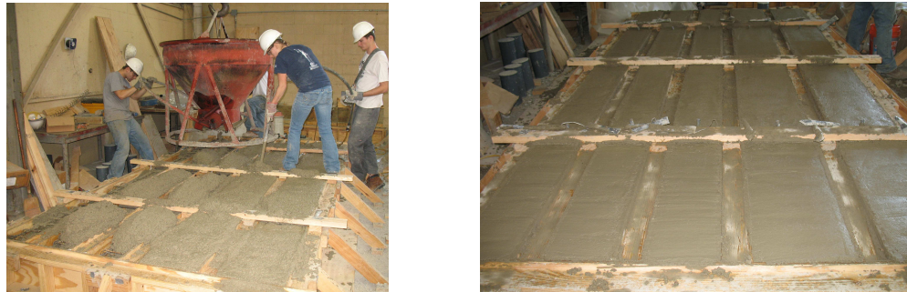
Figure 9: Placement of Concrete and Freshly Finished Beams
